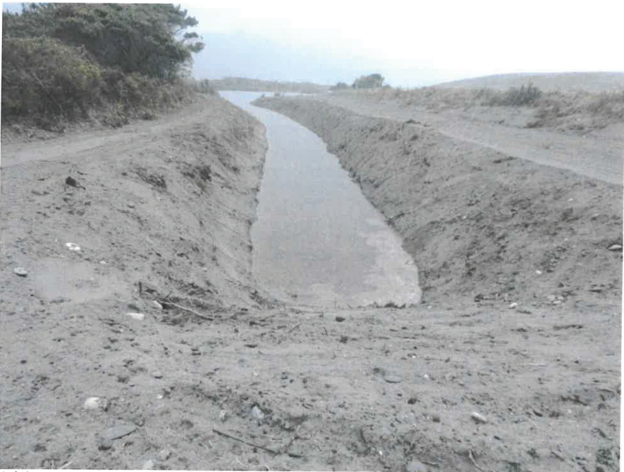
Cobden cut excavated to levels advised by River Edge Consulting.
