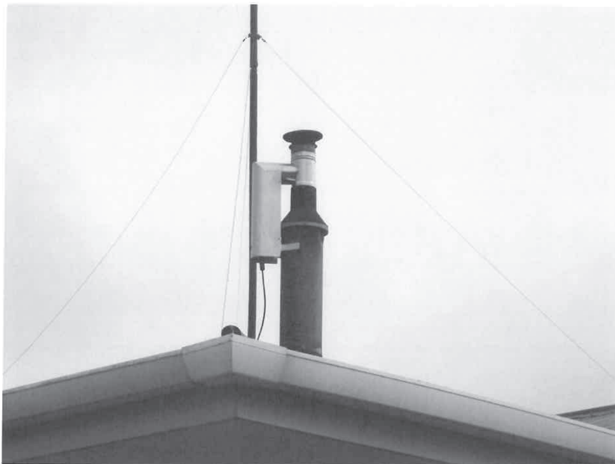
Oeko Tube device installed in Reefton
